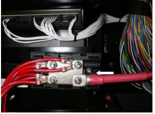
Unfasten the nut in the picture to remove the connection box.
